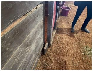
Image 4: Gap visible due to no door stop at bottom of sliding door in permanent barn
