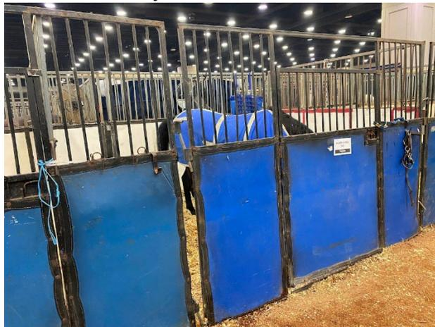
**Image 14: Gap between stall partition, North Wing**
