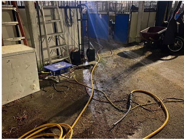
**Image 12: Electrical box at the back of Tent A adjacent to wet area**
